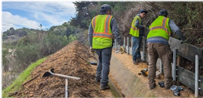
Installation of new retaining wall after clearing v-ditch
