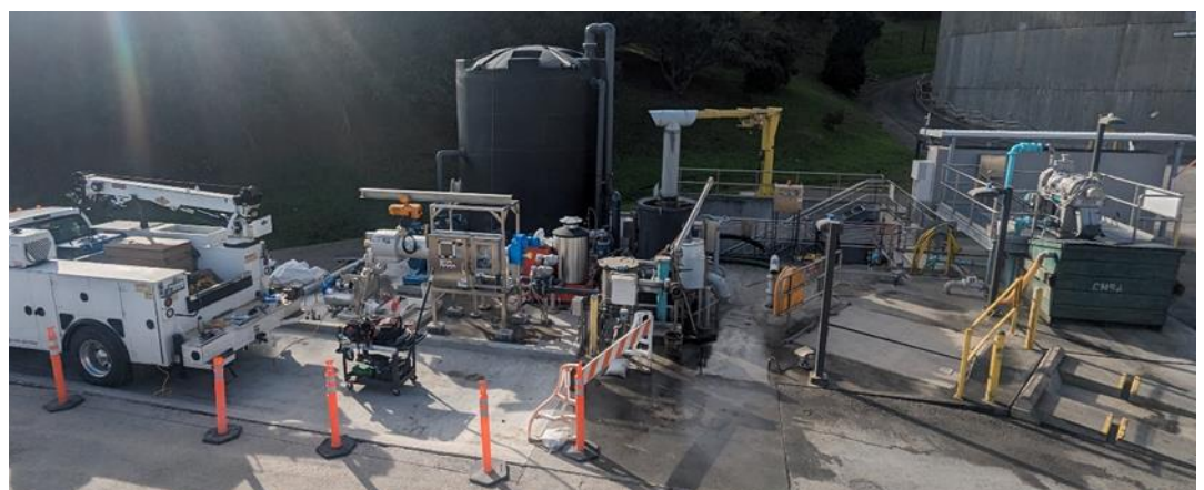
Construction at the new organic waste receiving tank near completion
